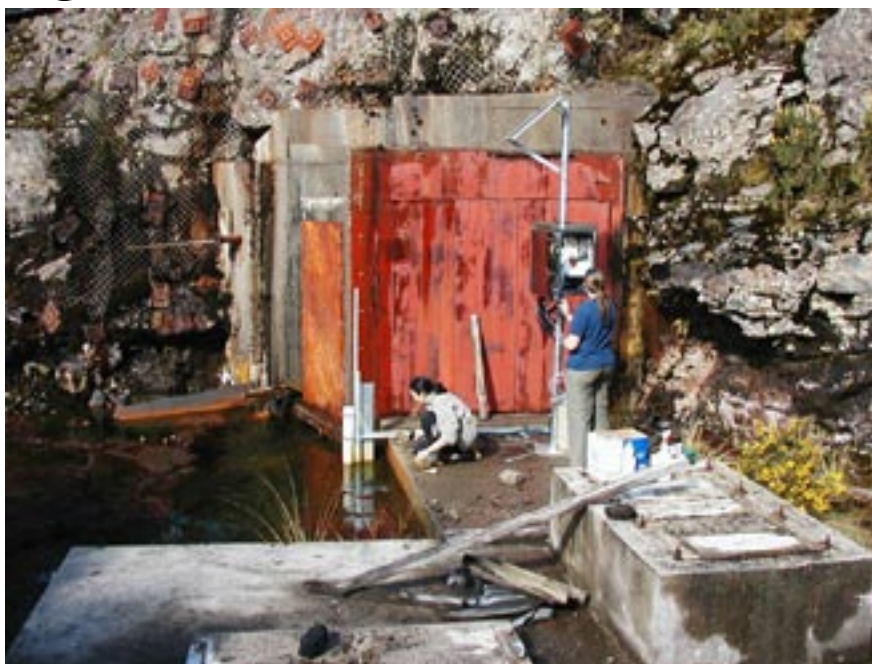
Members of the CRL Energy project team take acid mine drainage samples at the abandoned Sullivan Mine near Westport.
