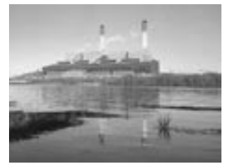
The Huntly Power Station runs largely on coal, is 1000MW, and has four large generators. The future could see more efficient coal-fired power plants to help secure New Zealand's energy supply.
